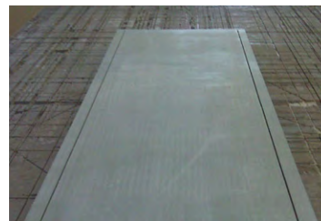
FIGURE 8 Saw kerfs for rodding.
