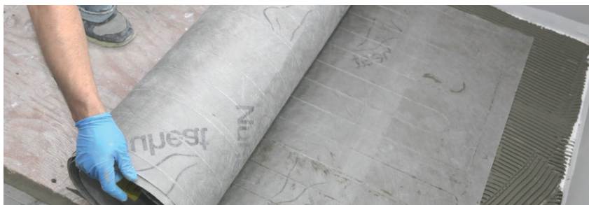
FIGURE 2.13: Place mat onto fresh thinset
