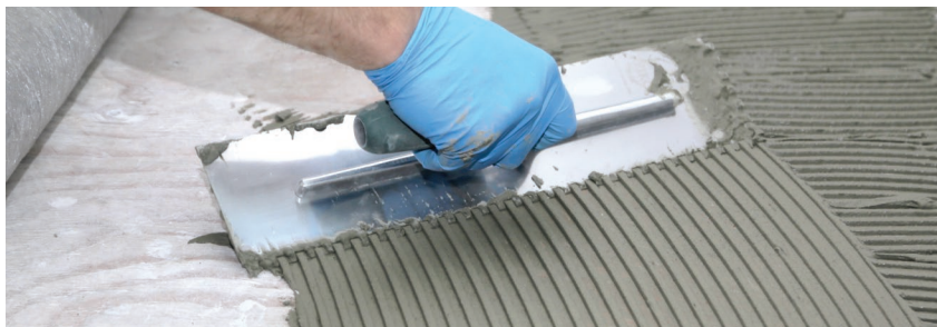
FIGURE 2.12: Spread thinset onto subfloor
