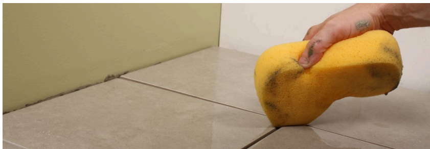
FIGURE 2.23: Clean grout lines
