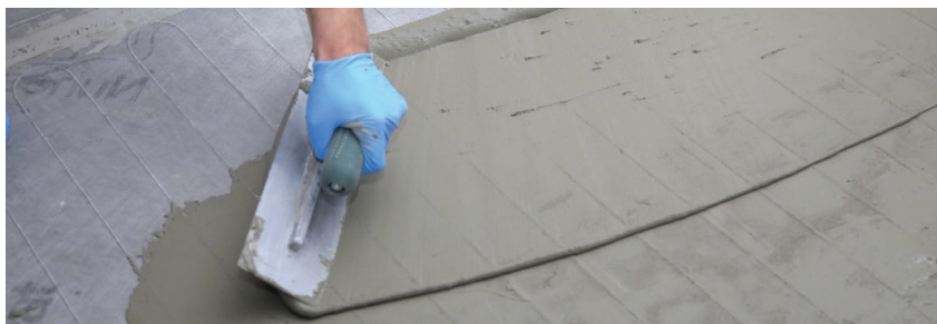
FIGURE 2.21: Install tile/stone flooring
