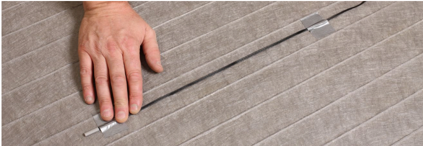
FIGURE 2.16: Secure floor sensor probe
