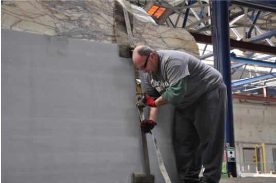
3. Once the slab is on the truck, the driver should secure the slab using at least two vertical straps to help evenly distribute the pressure along the slab. Tighten the straps just enough to restrict movement of the slab during transportation. Any excess tightening may lead to cracks.
