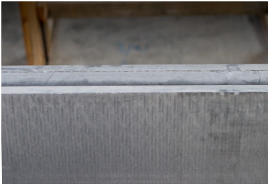
6. Place the third slab with the polished face against the polished face of the second slab. The unpolished face of the third slab will face out. Ensure that the bottom edges of slabs are touching. Unload all the slabs following this procedure.
